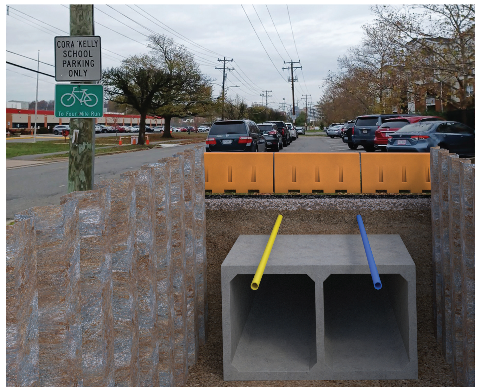
Two 8' x 7' box culverts will be installed on the east side of Commonwealth Ave
